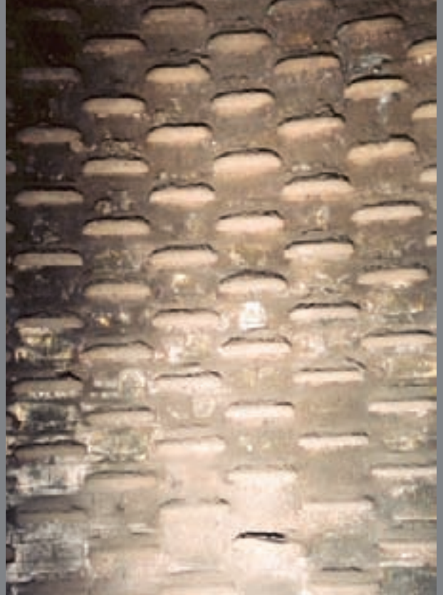
Corus IJmuiden No. 6 in 2002 after 16 year campaign No repairs required in shown area
