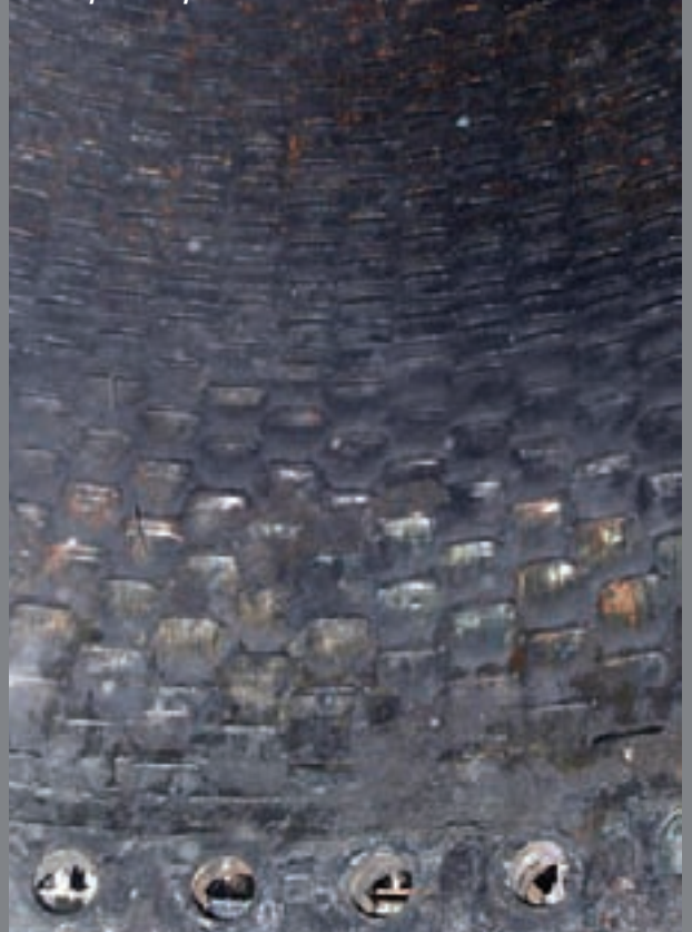
Corus IJmuiden No. 7 in 2006 after 15 year campaign No repairs required in shown area
